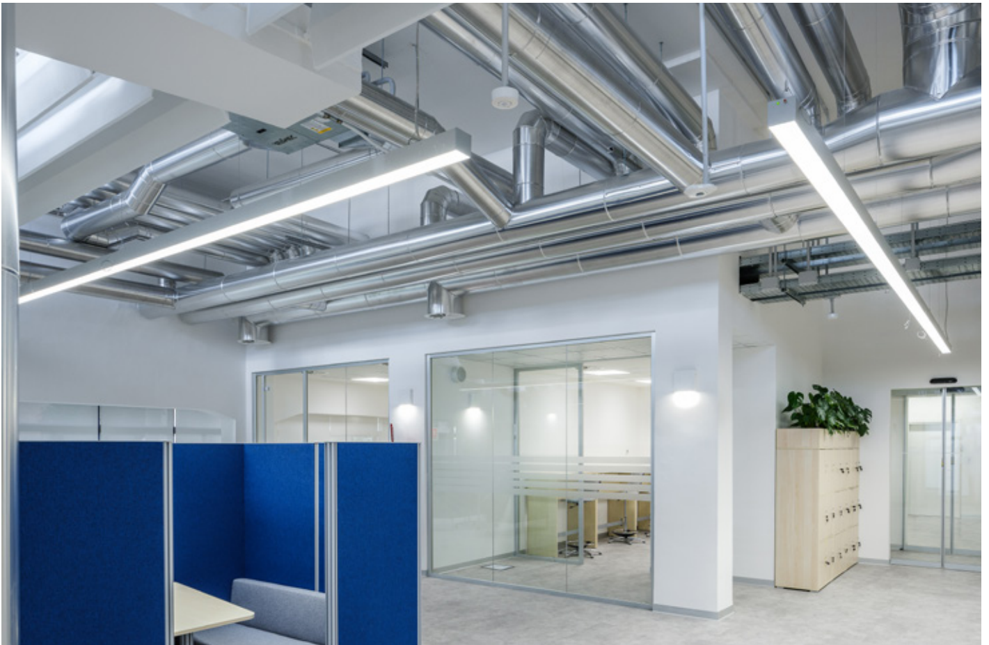
Offices comprensorio Olivetti | Naples | Italy
