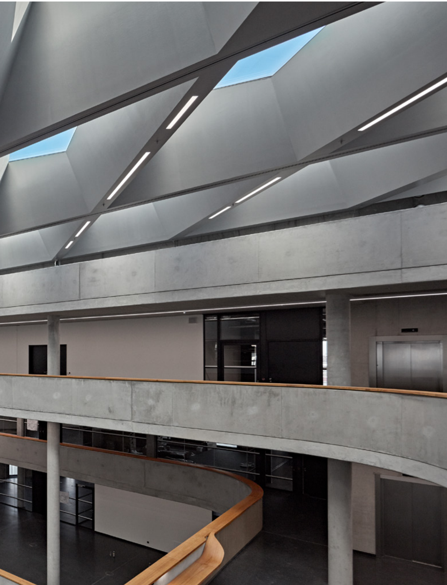
Zalando headquarters | Berlin | Germany
